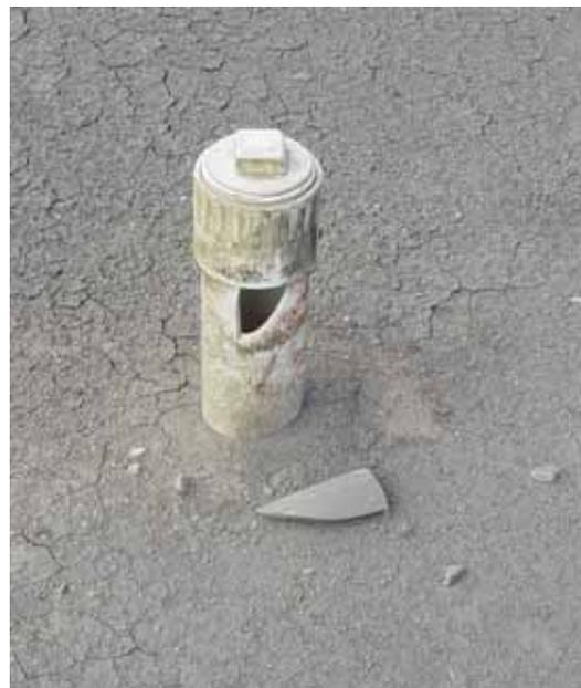
Broken cleanout pipe in sand filtration unit
