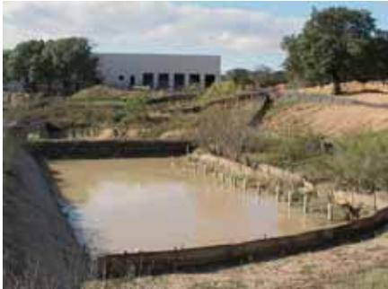
The photograph to the left shows that the sand filtration basin for a Sam's Club was clearly overloaded with sediment during construction.
